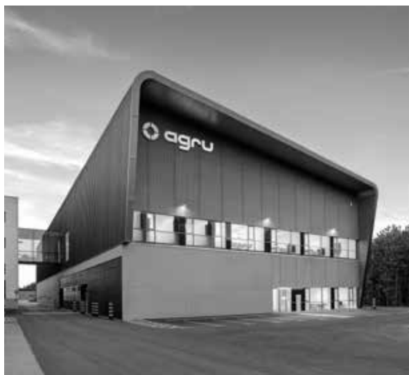
Figure B.1: New AGRU cleanroom plant.
